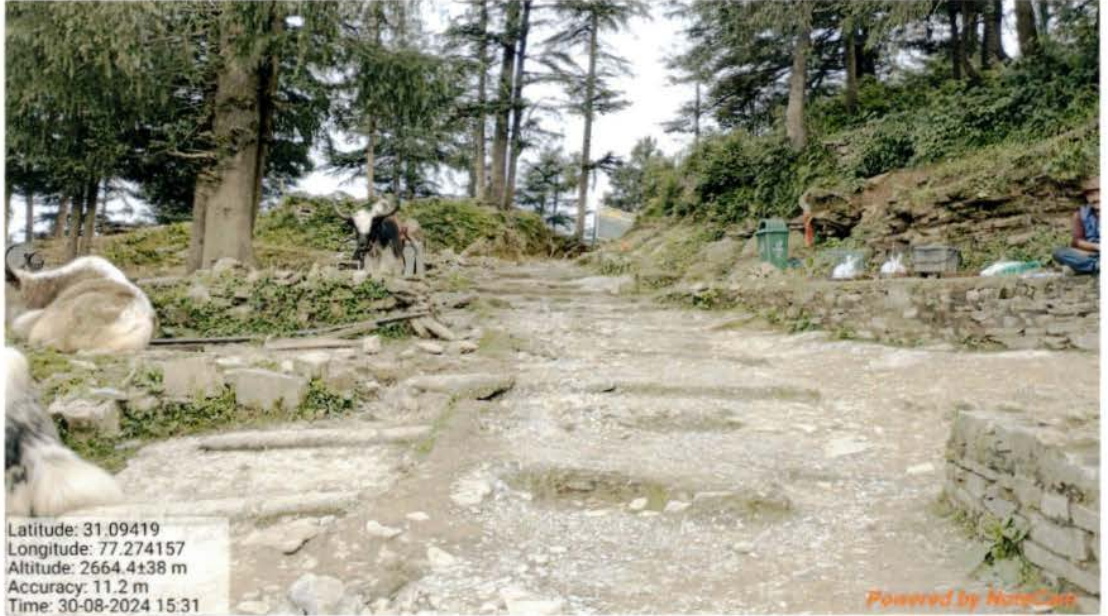
(Walking Trail) Before start of work
