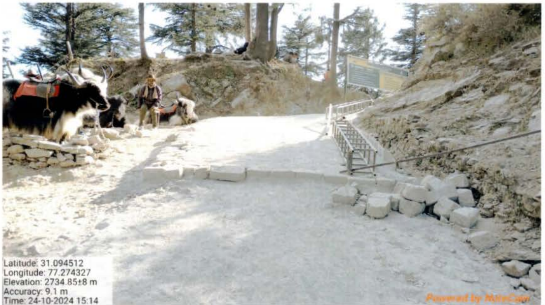
(Walking Trail) Work in progress
